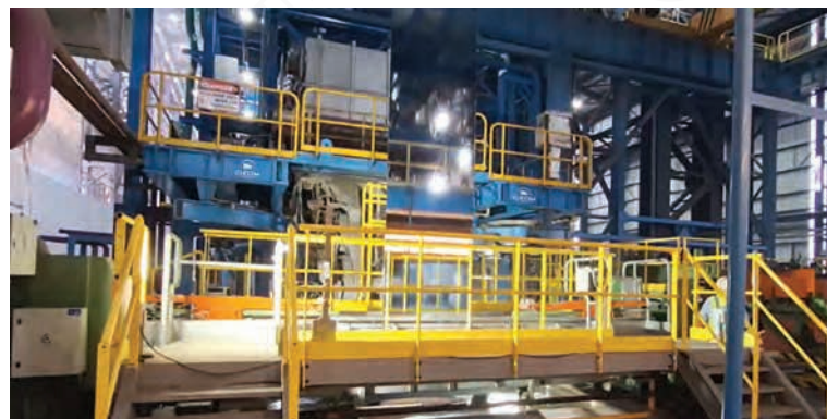
AM/NS Galvanization Continuous Line CGL#4, Hazira, India
